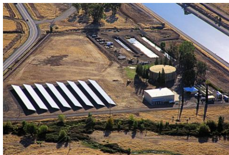
Thermalito Water and Sewer District’s Treatment Plant (535 Table Mtn. Blvd.)
